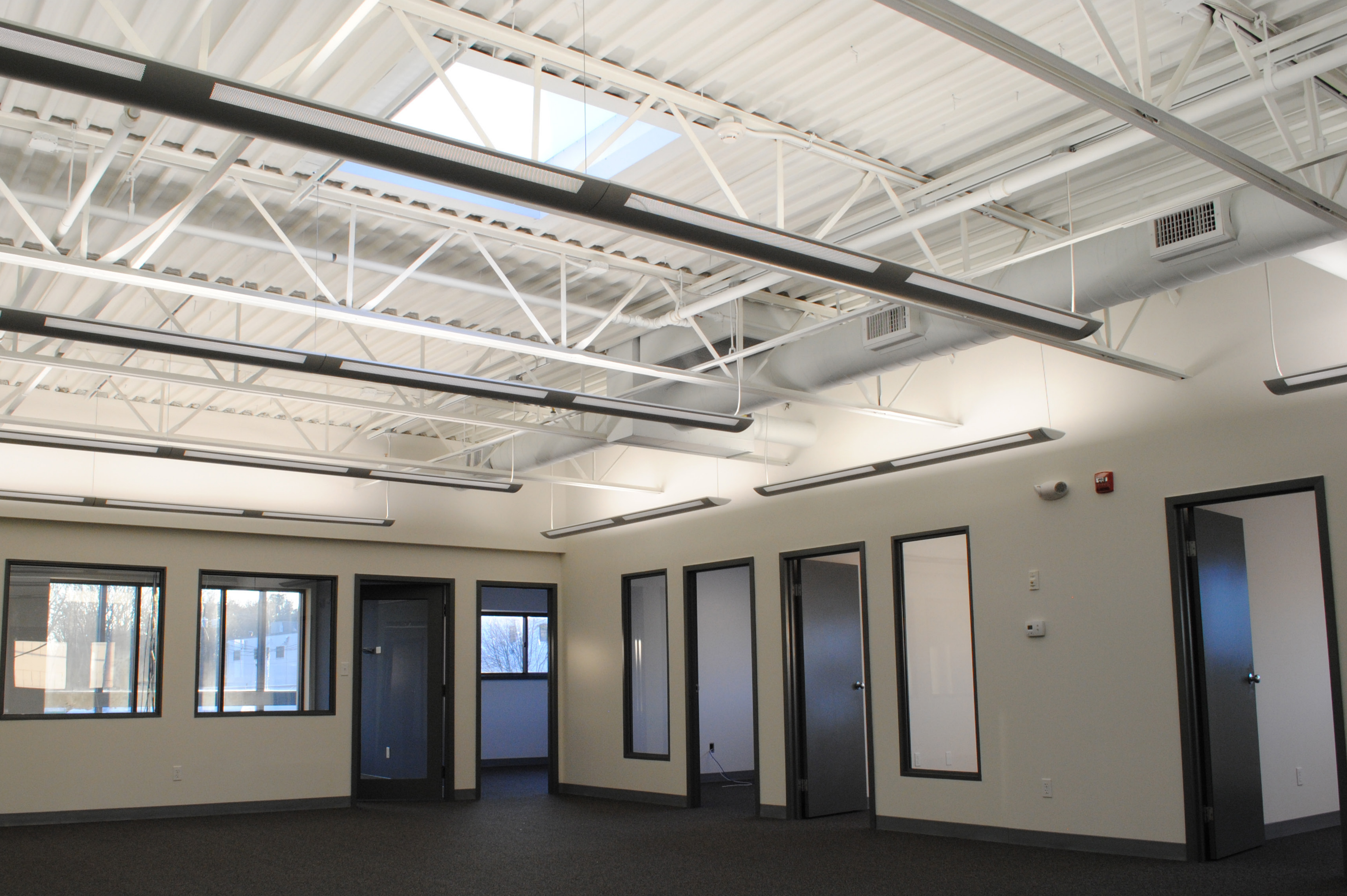
1 Merrill Street, Woburn
